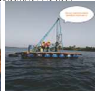
UNDER WATER DRILLING
