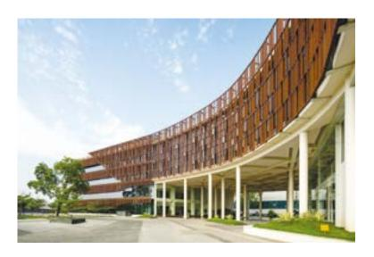
The project is designed to become a Net-Zero energy building. The balcony overhangs horizontally shade the southern façade. The façadeis designed with Low-E glass and aluminum fins on the East that are designed as per solar angles. The fins are designed to maximize views of the nearby hills and maximize daylight to the office areas while shading the direct sun. The combined setup reduces the energy requirement of the building by 20% from the base case of unshaded regular glass.
