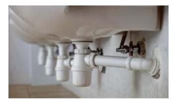
A drain pipe is any pipe used to transport water from one location to another. The primary goal is to discard sewage from homes, offices, and industrial areas. Water buildup can lead to flooding, significant damage, soil erosion, and other problems if disposed of improperly and inefficiently. As a result, drain pipes can be used on the job site and in the finished project.
