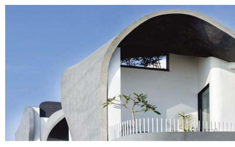
The superior volume of the structure has been broken down into more slender curves that allow abundant sunlight to enter the structure. It also facilitates adequate air flow and ventilation. Jutting concrete volumes provide shade for the openings and give shape and style to the overall facade.
