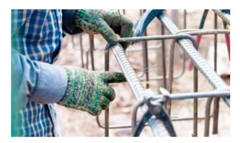
In construction, stirrups are used to reinforce concrete structures. They prevent the concrete from cracking under pressure while also offering strength and stability. Stirrup is a closed loop which is responsible holding the reinforcement bars together while constructing structures, such as columns and beams. They give the structure better lateral support, further improving its longevity and structural strength.
