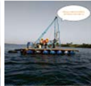
UNDER WATER DRILLING
